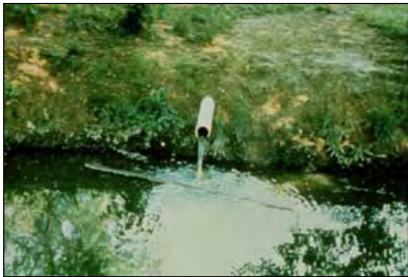
Figure 2: Direct Discharge from a Straight Pipe
