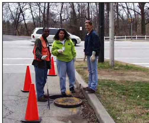
Figure 54: Traffic cones divert traffic from manhole inspection area
