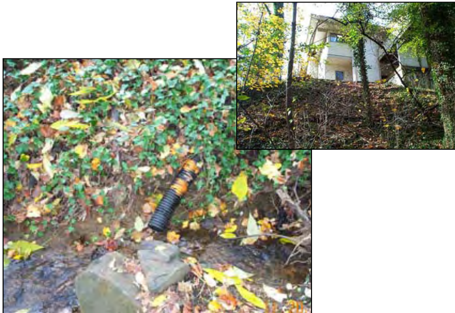
Figure 25: The origin of this corrugated plastic pipe was determined to be a roof leader from the house up the hill.
