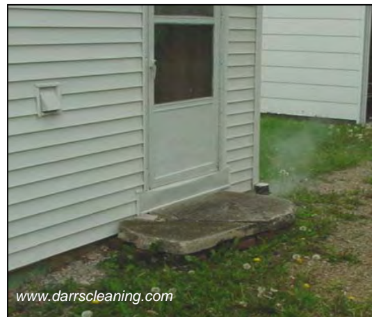
Figure 71: Smoke Rising from Sewer Vent
