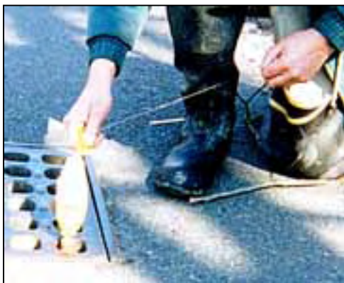
Figure 60: Optical Brightener Placement in the Storm Drain
