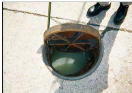
Figure 55: Manhole observation (left) indicates a sewage discharge. Source is identified at an adjacent sewer manhole that overflowed into the storm drain system (right).
