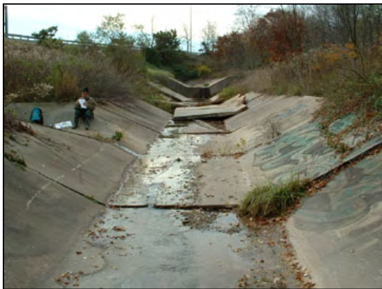
Figure 19: Walk all streams and constructed open channels
